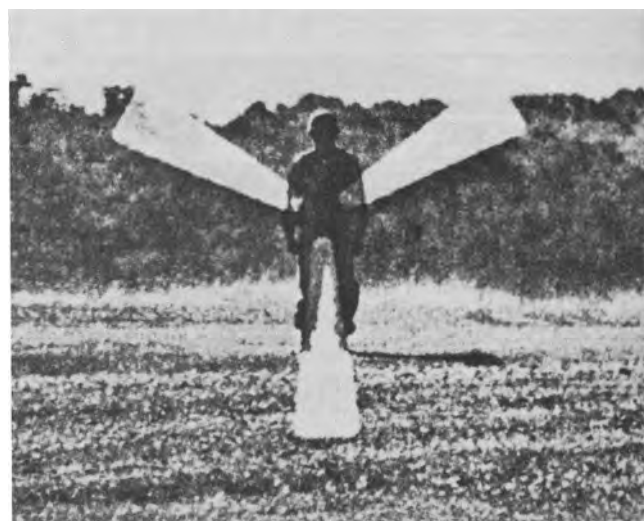
303. The final RCS reticle design, which was projected as an illuminated, inverted yellow "Y" onto the target. Not adopted.
