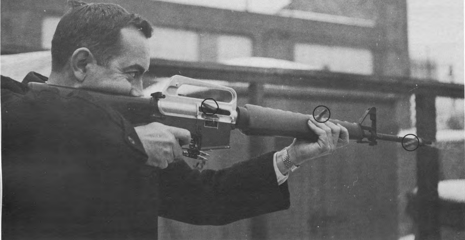
175. Colt designer Rob Roy firing the original, regular-barreled belt-feed rifle shown in fig. 174. Note the three circled empties, and the links of the disintegrating belt exiting through the link ejection port.
