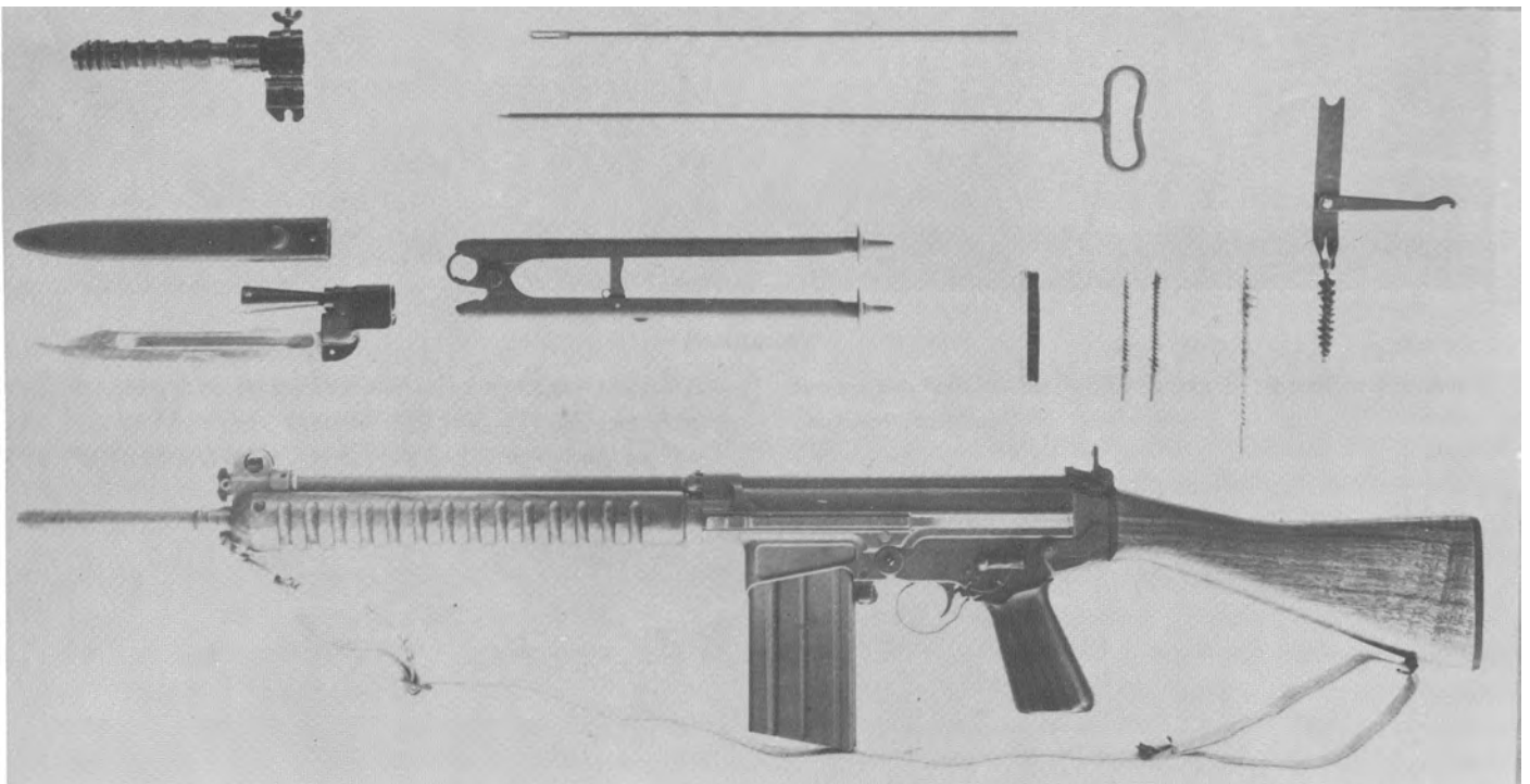
2. An early "Lightweight Automatic Rifle" from Fabrique Nationale of Belgium, shown with a rare array of proposed accessories. Also used at Fort Benning and Aberdeen in 1950. Caliber .280/30. QAD (Ord) Pattern Room
