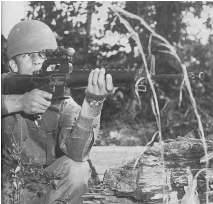
298. One of the sixty-odd sighting systems evaluated in the Frankford Arsenal sight enhancement project of 1967-75. The British "Singlepoint" sight was originally developed in 1968 for UK trial on L1A1 rifles. Not a true see-through sight, the Singlepoint offered improved target acquisition and hit capability by projecting a bright red aiming dot onto the target, which was viewed with both eyes open.
